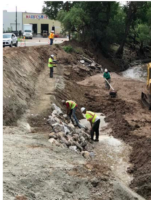
Second Repair of IOI Exposure
