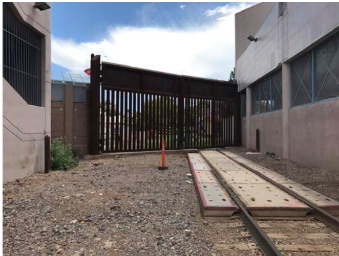
Concrete poured around tracks offers a safer environment for the officers
