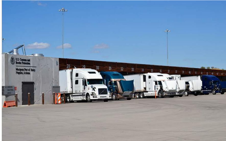
Mariposa Port of Entry in Nogales, Arizona. (Photo by Andrea Jaramillo Valencia/Cronkite News)
