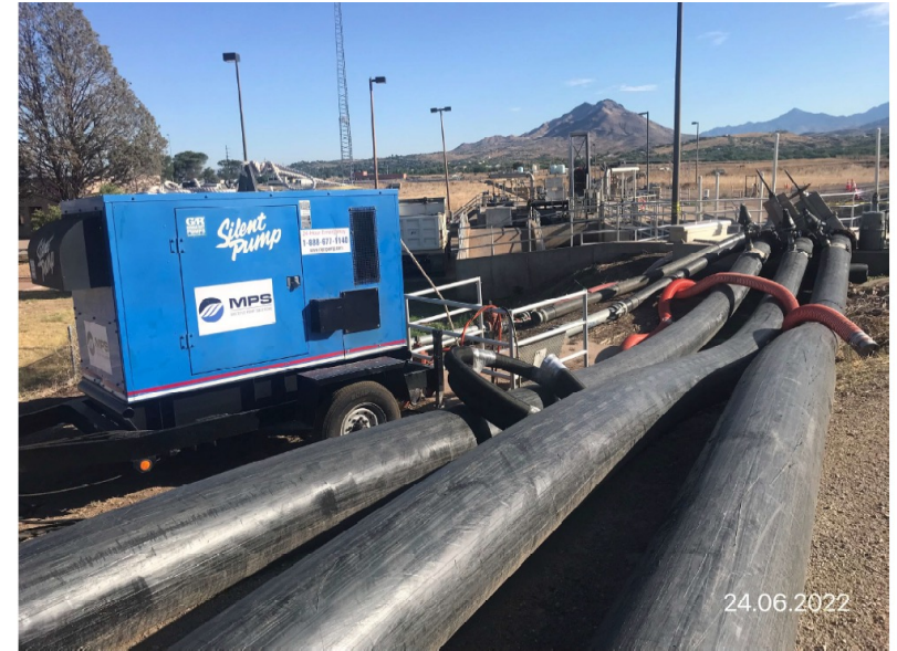
Sewer bypass HDPE pipe and pumps
