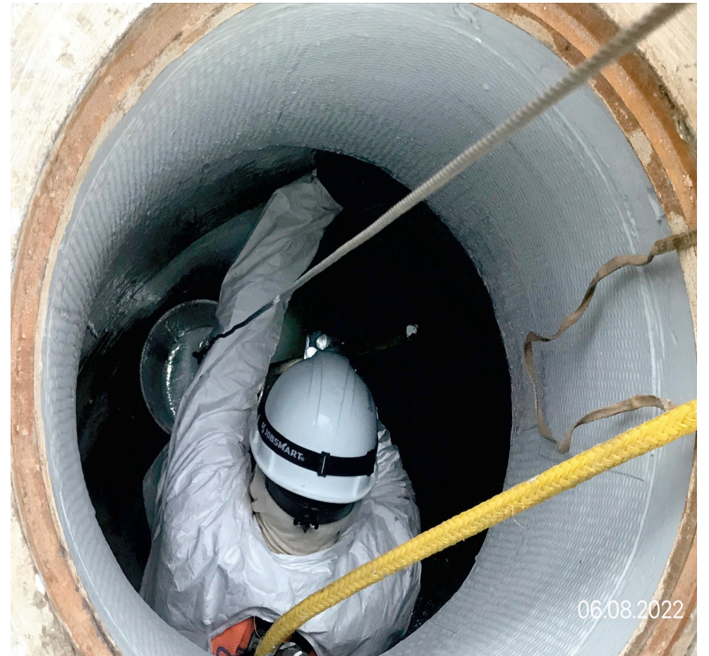
Top Coating of MH87
